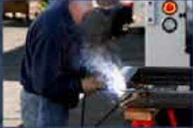
Onsite Welding Repair
